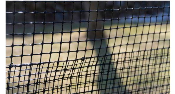
Here is how the top of your fence will look when it is complete. Note how the top of the fence only has the polypropylene mesh on top (to prevent climbing).
